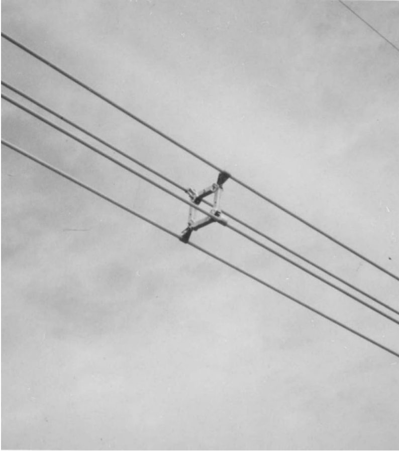
Figure 6.16. Spacer in four-bundle power line.
